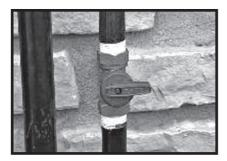
When you've finished checking the gas pressure, close the manual shutoff valve.
